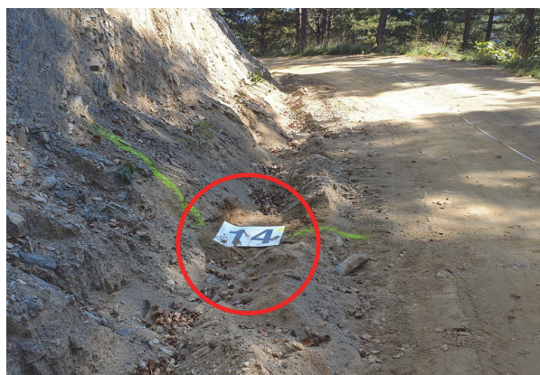
Figure 3. Installation of check point.
