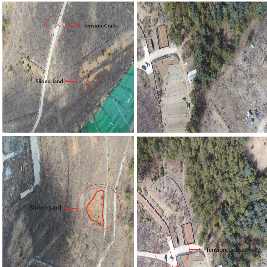
Figure 8. Landcreep area analysis results using drone image. Note: The ocher color inside the red line is where the collapsed area was formed by landcreep.
