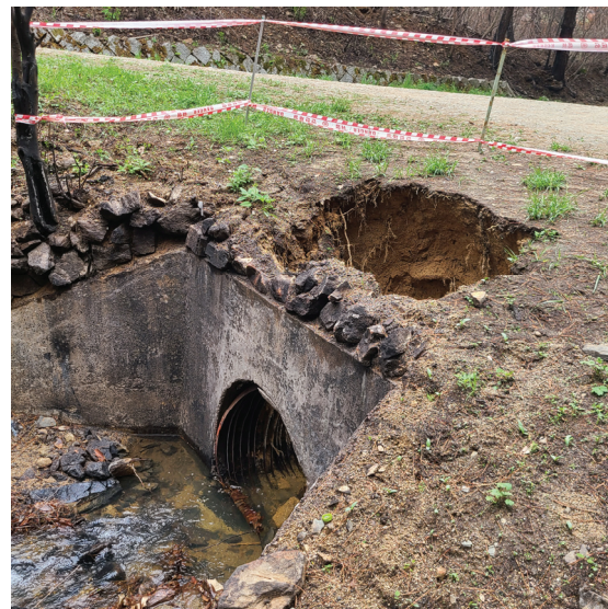
Figure 1. Damage to wing walls and culverts caused by forest fire (Seo-gu, Daejeon-si).
