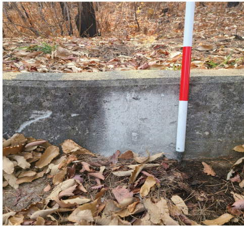
Figure 6. The strength of forest fire damaged and undamaged retaining wall in forest road ( p < 0.001 ).
