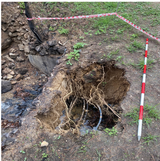
Figure 1. Damage to wing walls and culverts caused by forest fire (Seo-gu, Daejeon-si).
