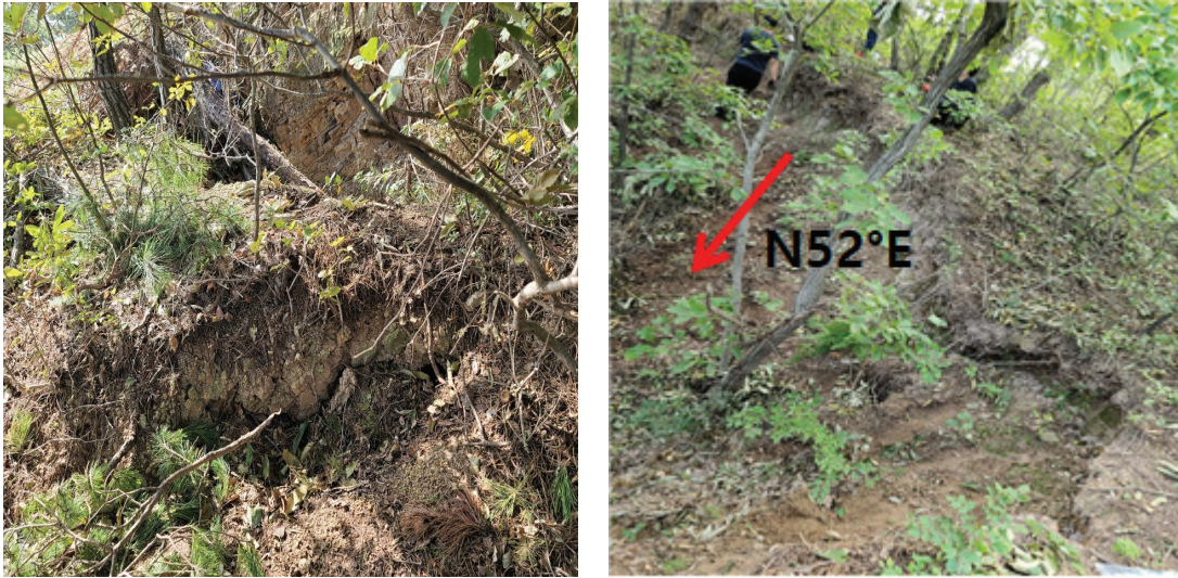
Figure 8. Tension crack caused by landcreep.
